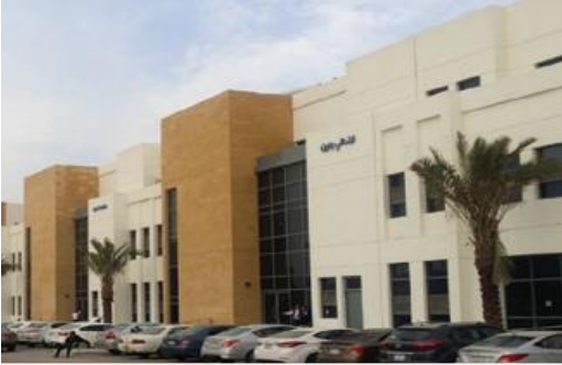
Dar Al Baraa School
