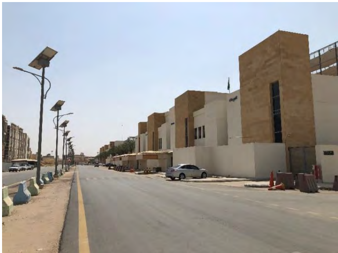
Source: JLL Inspection 2022
