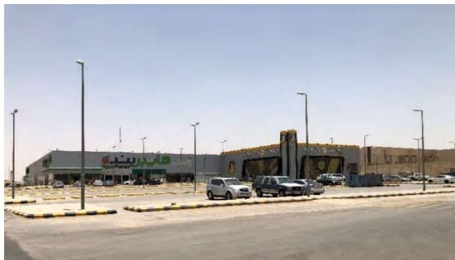
Source: JLL Inspection 2022
