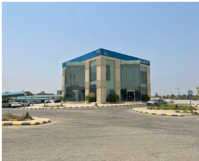
Source: JLL Inspection 2022
