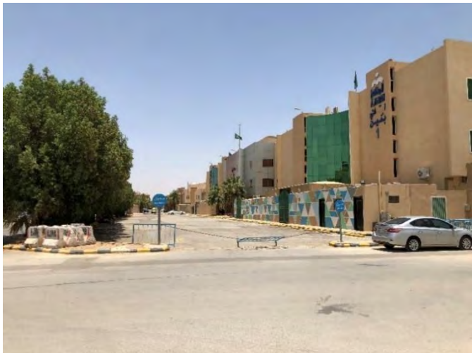
Source: JLL Inspection 2022
