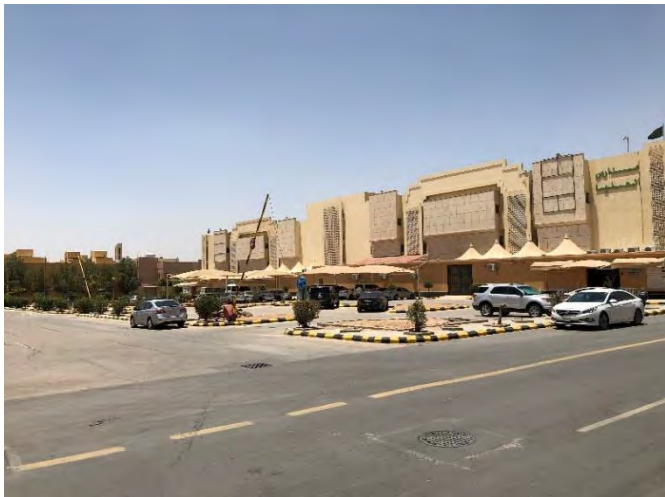
Source: JLL Inspection 2022
