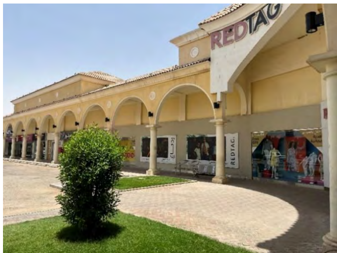
Source: JLL Inspection 2022
