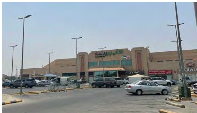
Source: JLL Inspection 2022
