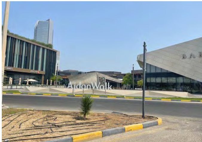
Source: JLL Inspection 2022
