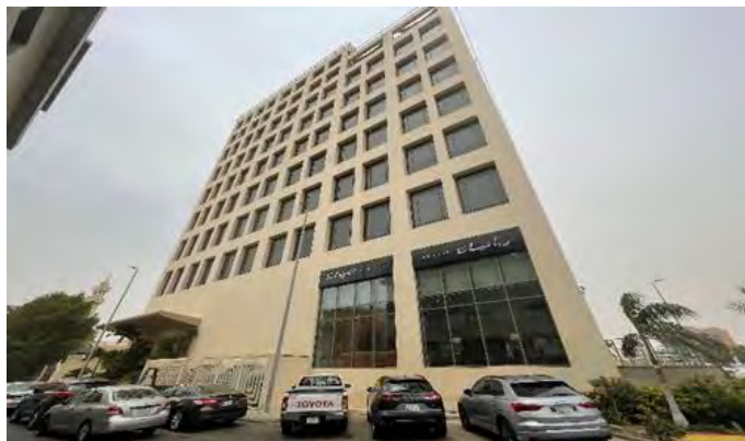
Source: JLL Inspection 2022
