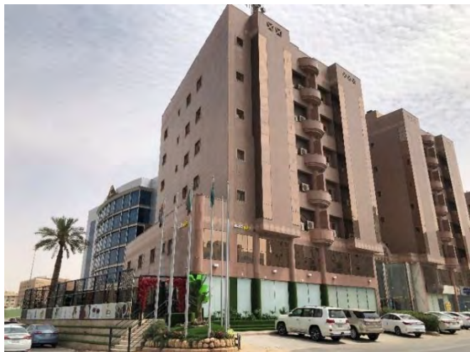
Source: JLL Inspection 2022
