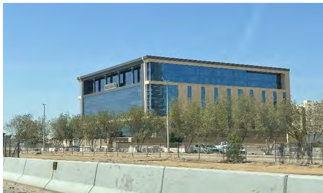
Source: JLL Inspection 2022
