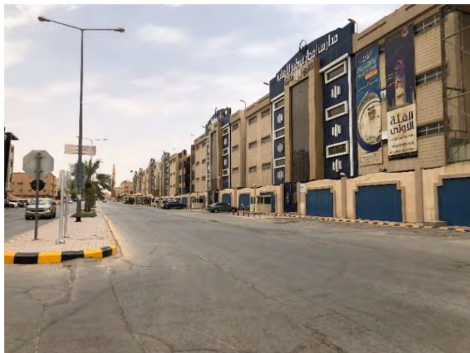
Source: JLL Inspection 2022
